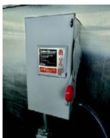
Combi-Duo Unit Independently Fused Power Supply Line
