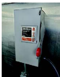
Combi-Duo Unit Independently Fused Power Supply Line
