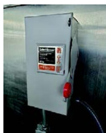
Single Unit Independently Fused Power Supply Line
