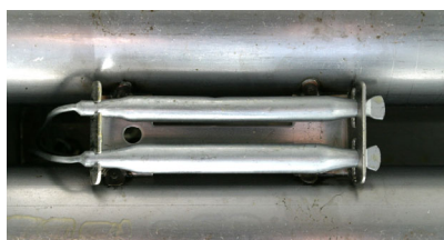
Typical high-limit/sensor probe locations and mounting hardware.
